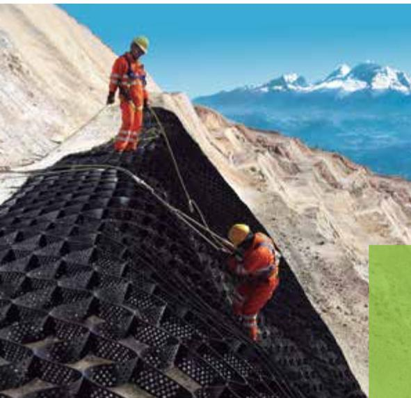
Designed for additional stability by integrating tendons on steeper slopes or when a geomembrane or hard soil/rock surface prevents anchoring with stakes.
